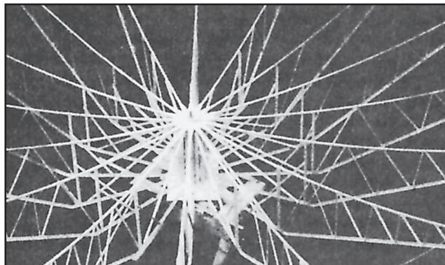
**Fig 29**—Detailed look at the hub assembly for the ZL1BJQ dish. Most of the structural members are made from  $\frac{3}{4}$ -inch T section.
