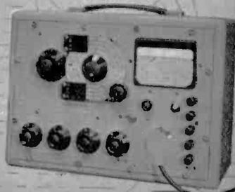
vision receiver shown by this firm. There are four R.F. stages in the vision channel with the first common to the sound channel. It includes a 9-in magnetic-type tube and derives its E.H.T. in a rather unusual manner by rectifying the output of an R.F. oscillator. Extensive use is made of miniature valves.
